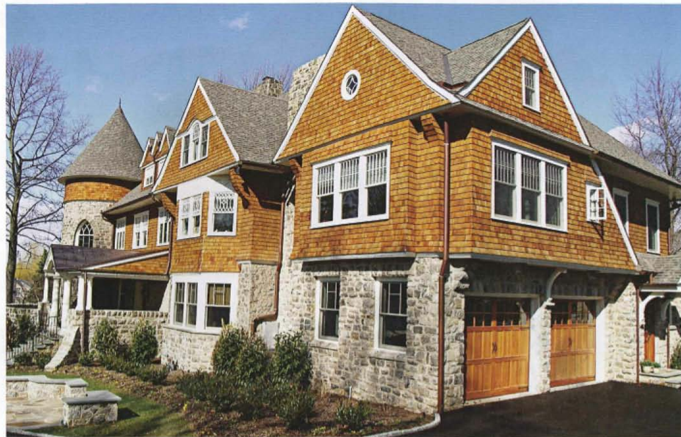
By carefully dismantling the home's former arched stone entryway, the Gardner/Fox team was able to power-wash the stones and use them to match the exterior on most of the two-and-a-half car garage addition.
